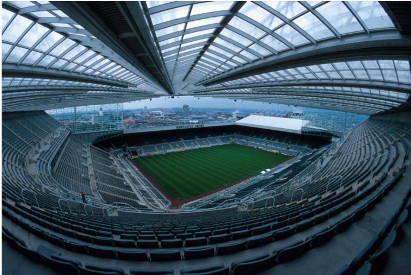
St James' Park in 2000. The new L-shaped roof is cantilevered to a dizzying depth of 65.5m, while at 60m tall at its highest point it is 1m taller than the Tyne Bridge.
