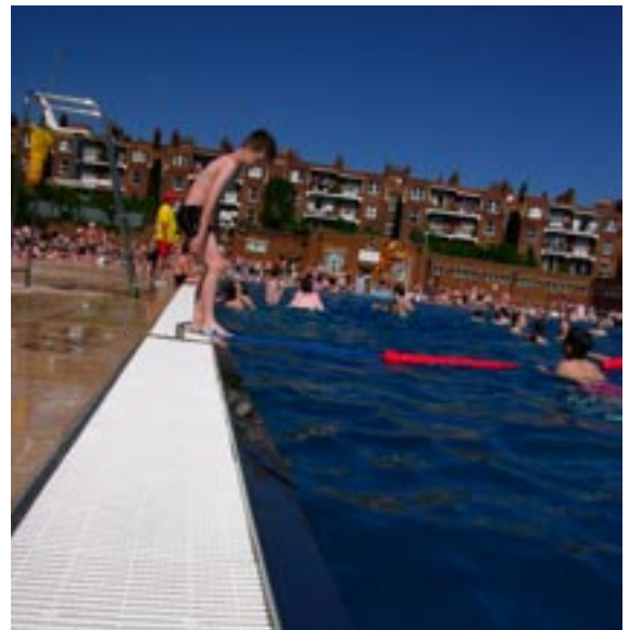
Parliament Hill Fields Lido viewed from the east ( above ), with the new deck level perimeter channel and stainless steel lining ( right )
